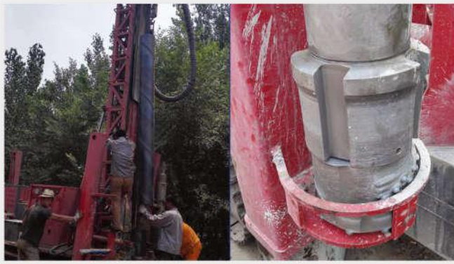
Water Well Drilling
