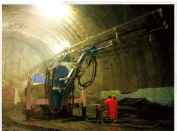
Pipe Roofing
